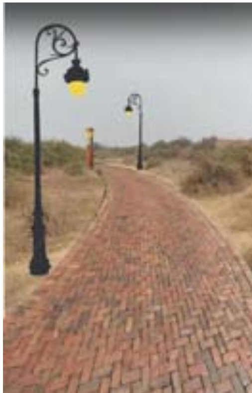
Figure 21: provision of brick on edge flooring to access the monuments.
