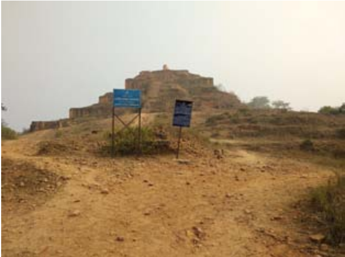
Figure 11: Current condition of the site
