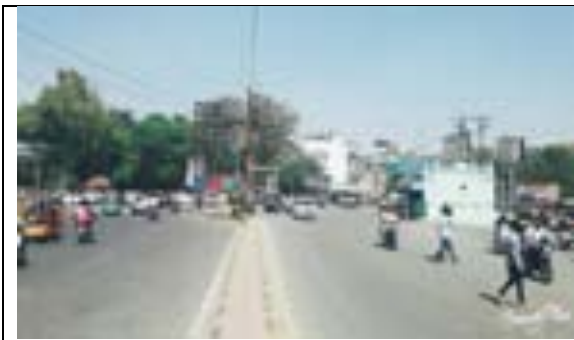
Figure 104: Existing Road condition at Chowki Chauraha
