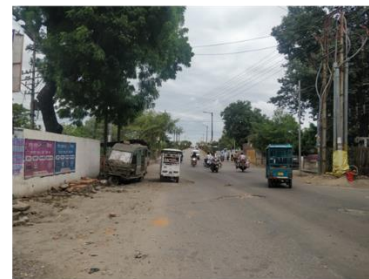
P1 Flyover Entry
