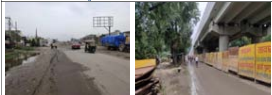
Figure 89: Flyover construction at Lal Phatak Railway Crossing
