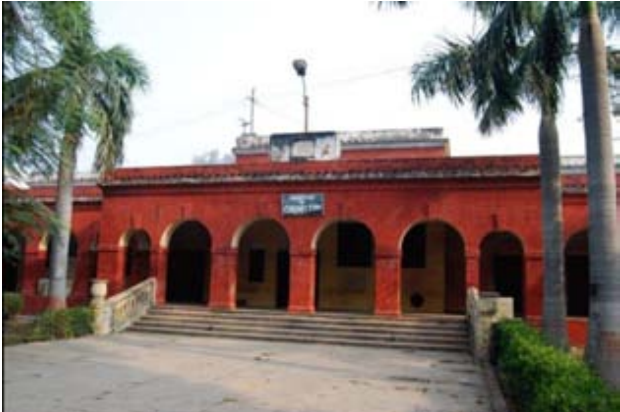
Figure 38: Current condition of chemistry department block
