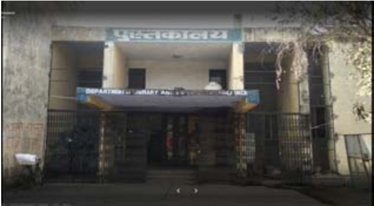
Figure 36: Image showing current condition of the library building
