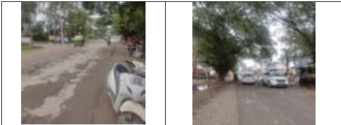
Figure 88: NH 530B near Circuit House road
