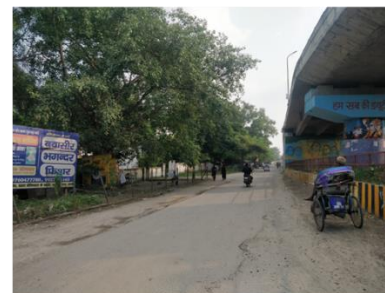
Road below Flyover
